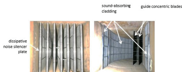
Fig. 2: The noise reduction complex in the flue behind the smoke pumps DOD-31.5FGM in front of the flue of the TGMP-314 power boiler
