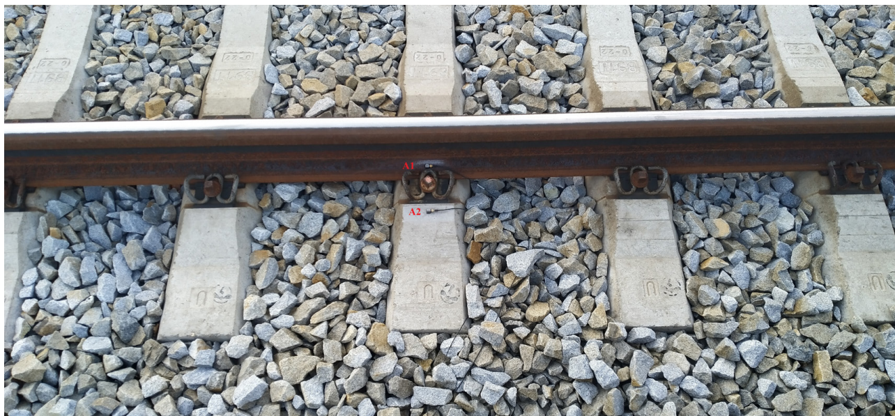
Fig. 3 The location of vibration acceleration sensors on the rail grid
